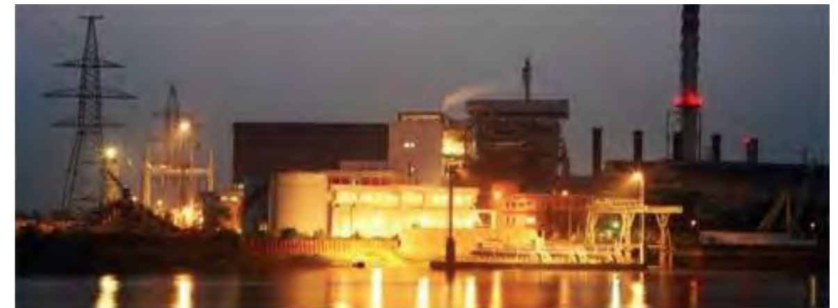
Ashuganj Power Station Co. Ltd. (First Simultaneous Heat & Cool VRF In Bangladesh)
