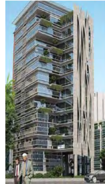
South Breeze Square, Proposed Platinum LEED Project
